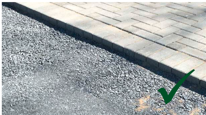
Installation height as specified.
