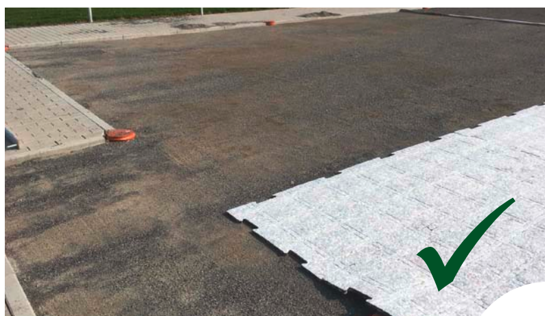
Gravel leveled and firmly compacted.
