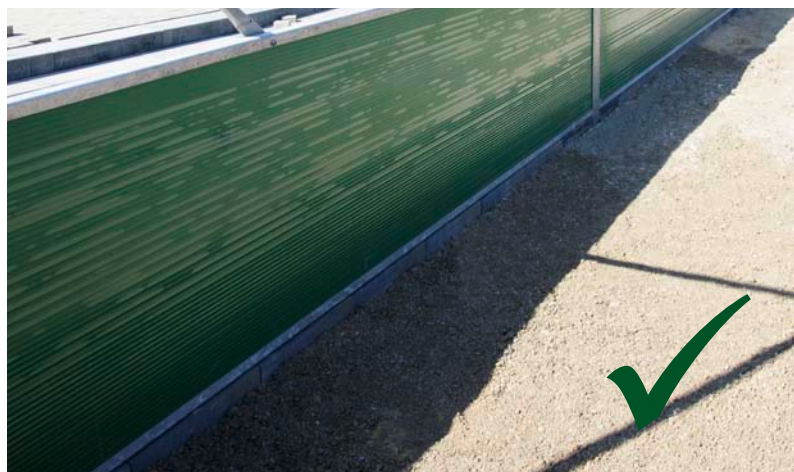
Curb placed correctly (inner edge flush with boards).
