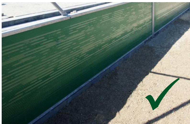
Curb placed correctly (inner edge flush with boards).
