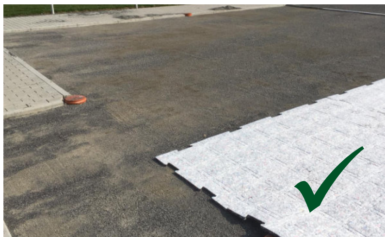
Gravel leveled and firmly compacted.
