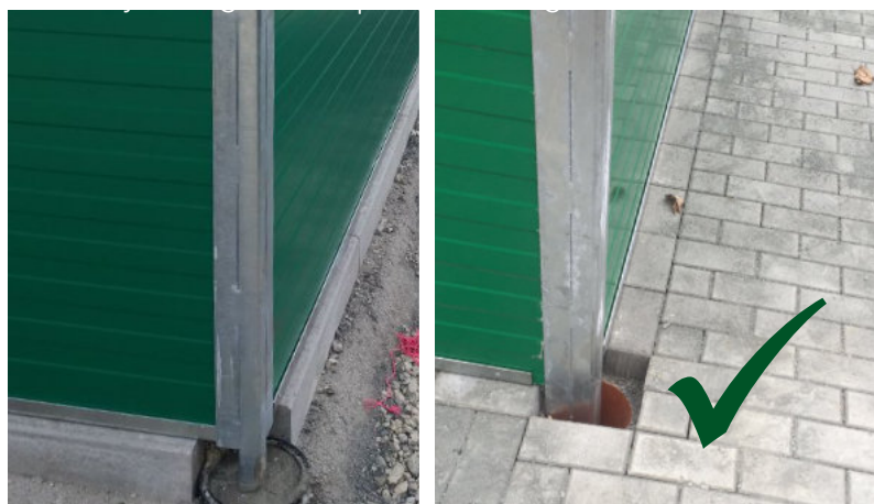
Accessible conduits, closed with lids if necessary, ideally aligned with the center of the curb.
