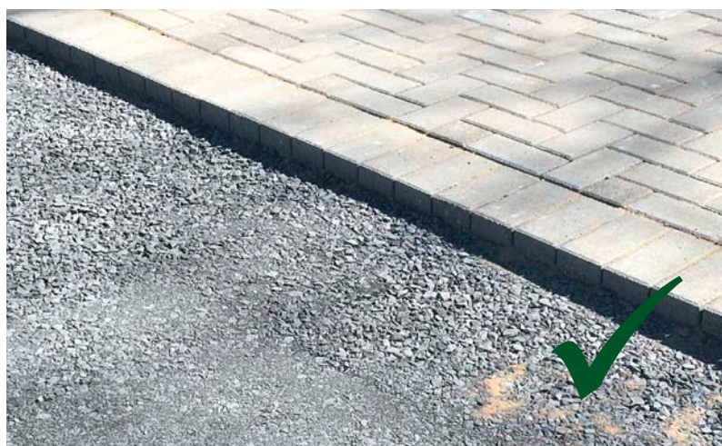
Even installation height, as specified.
