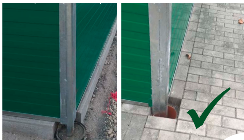
Accessible conduits, closed with lids if necessary, with the lid flush with the top of the curb.
