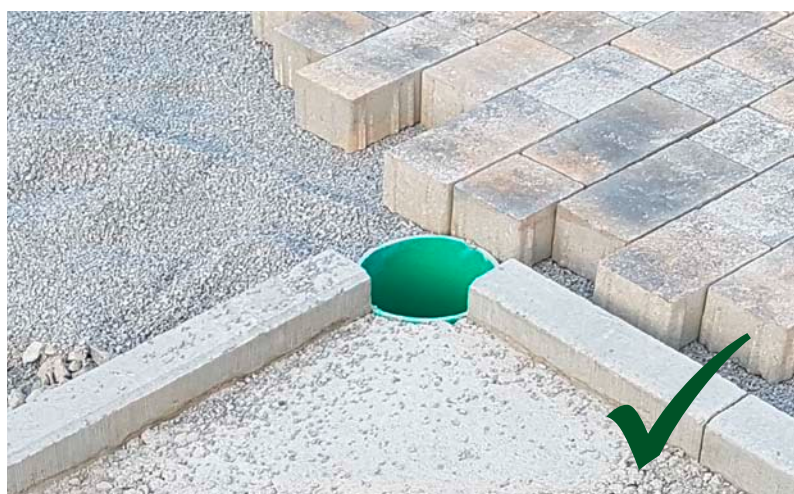
Foundations / conduits placed according to the foundation plan.
