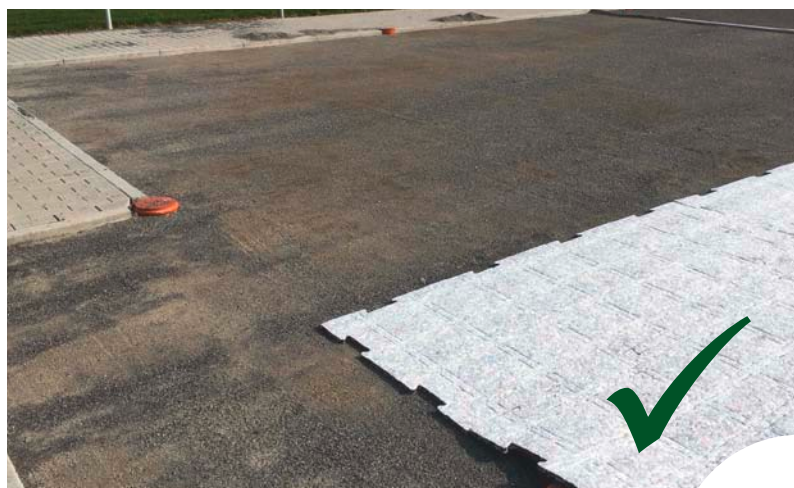
Gravel leveled and firmly compacted.
