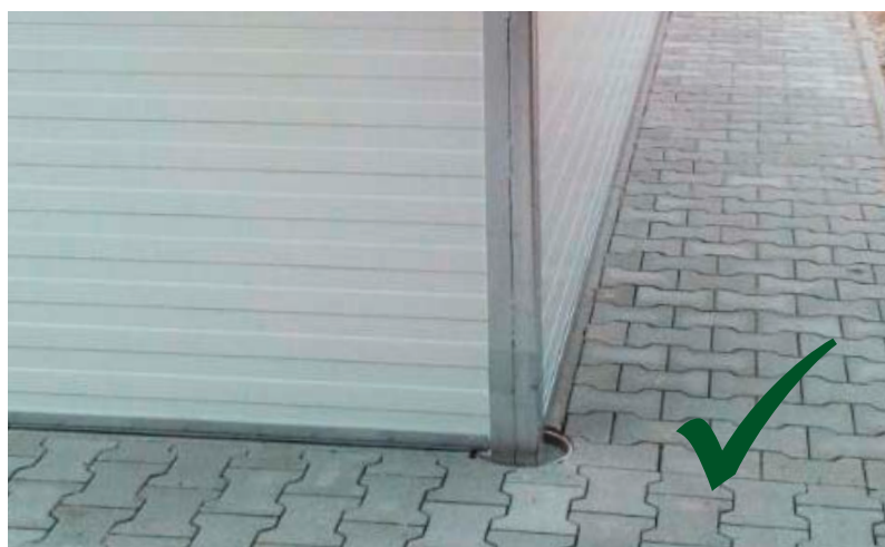
Foundations / conduits placed according to the foundation plan.
